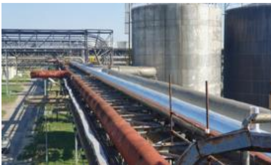
Views of the new P3 steam pipeline route on bridge C of DN 400
